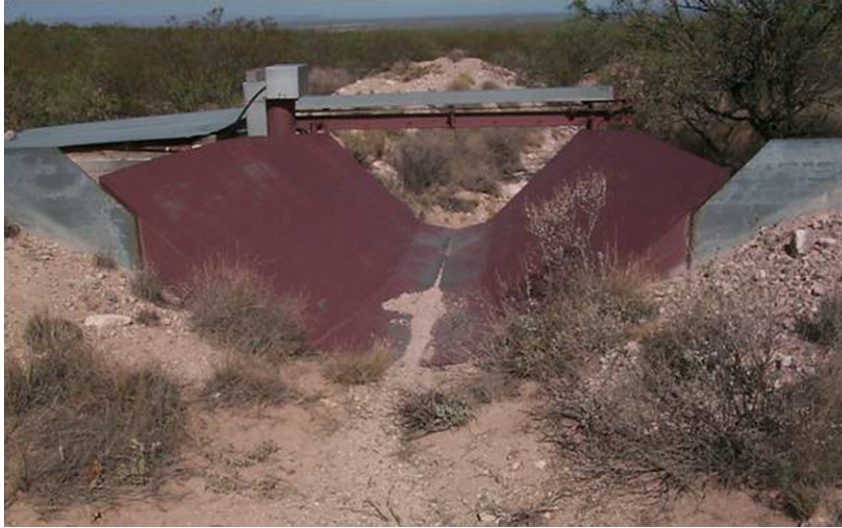
Fig. 3. The 2.8 \text{ m}^3 \text{ s}^{-1} Santa Rita flume where runoff from the catchment is measured (looking downstream).
